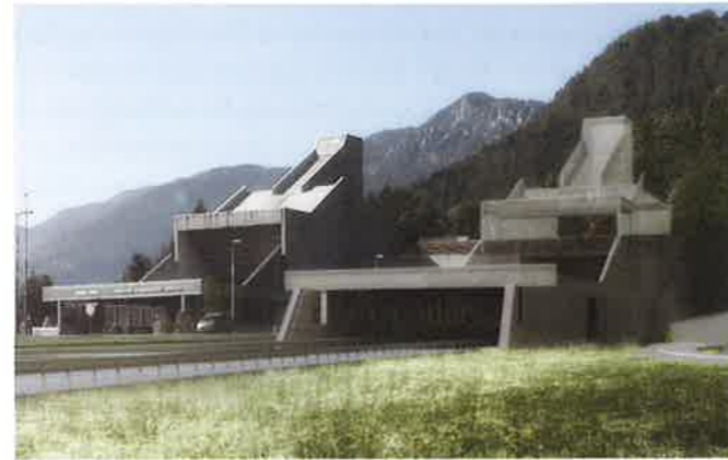
Ansicht Portal Karawankentunnel (© ASFINAG and DARS, Elea-ic)
